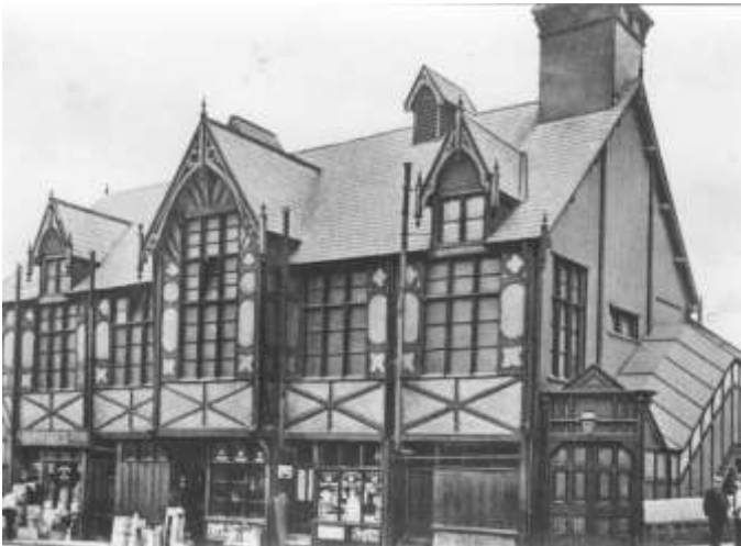
Fig: 50 Winsford Town Hall, c.1900
