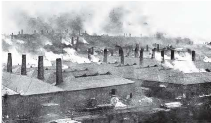
Fig: 74 Winsford's smoking chimneys
